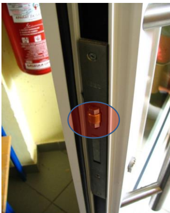
Inadequate lock on a fire rated door
