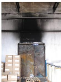
Non fire rated door – non exposed side
