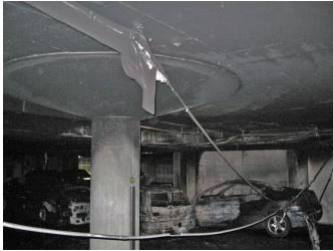
Significant damage on a smoke control duct – 30 minute fire resistance
